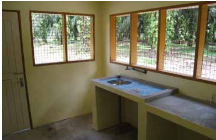
■ Housing - Refurbished Kitchen, Teja Estate
