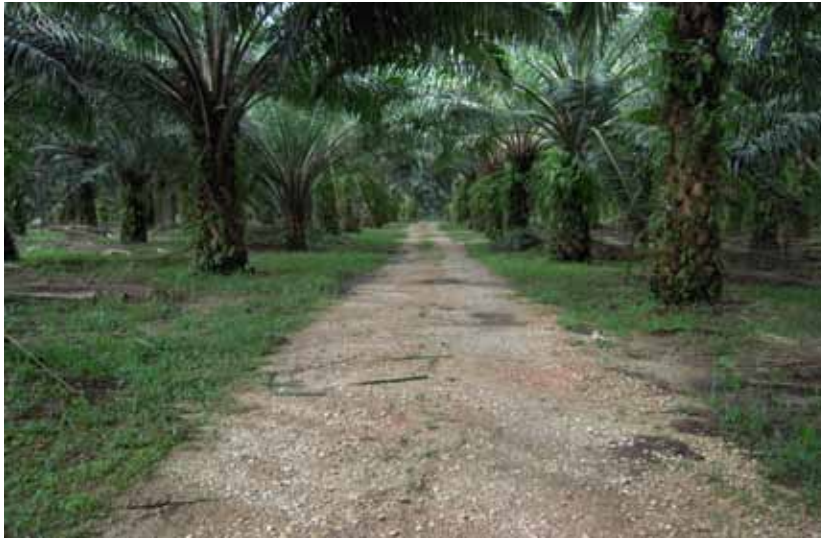
■ Roadworks - Upgrade Of Field Road, Buloh Akar Estate
