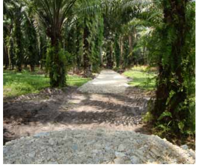
■ Roadworks - Upgrade Of Field Road, Teja Estate
