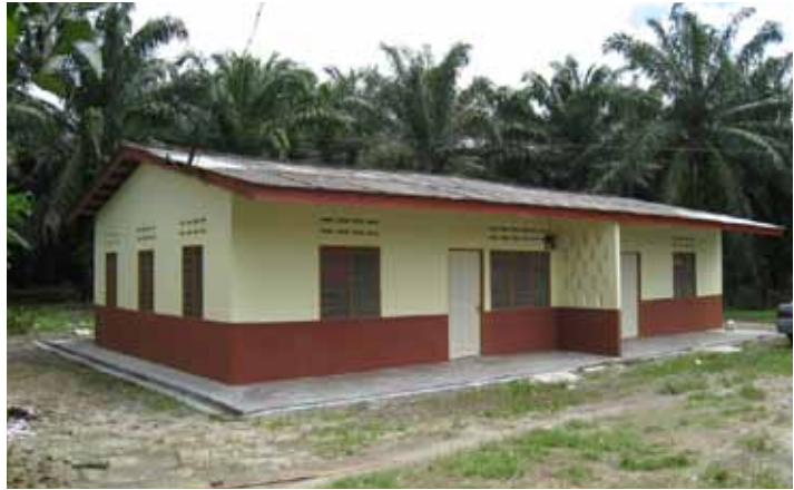
■ Housing - Refurbished Labour Lines, Teja Estate
