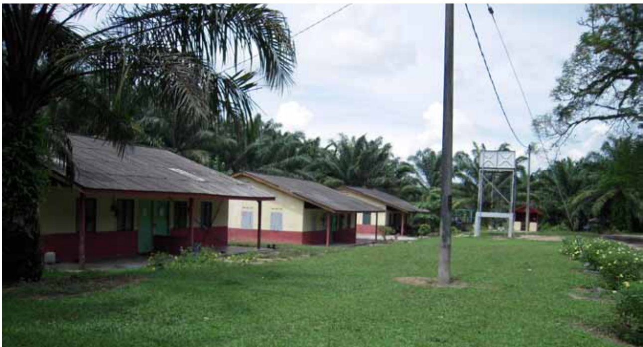
■ Housing - Refurbished Labour Lines, Chendrong Estate
