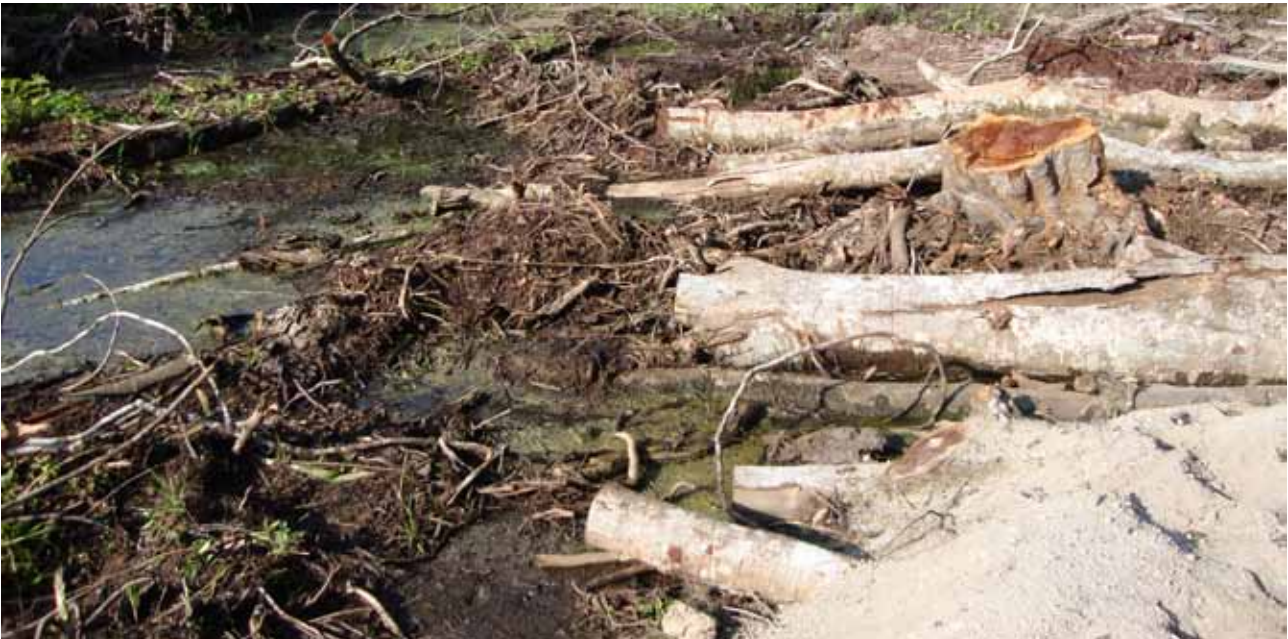
■ Teja Estate - Clearing Of Swamp
