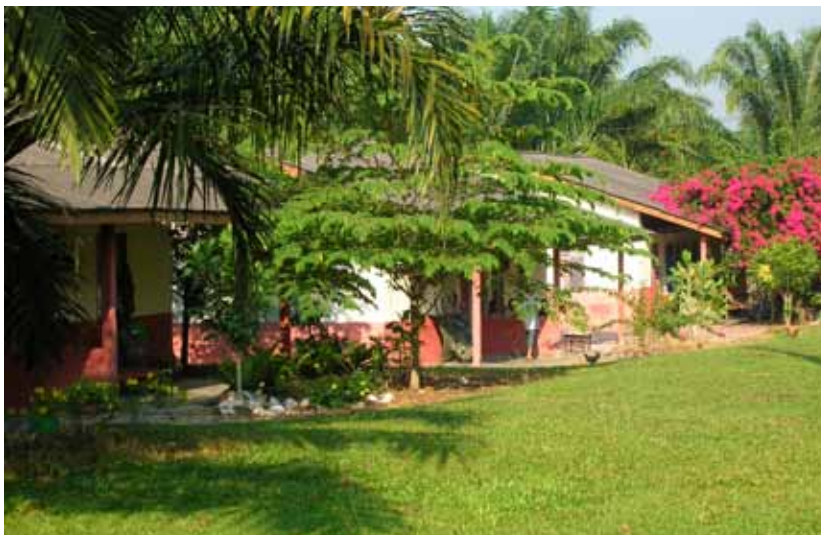
■ Housing - Refurbished Labour Lines, Narborough Estate
