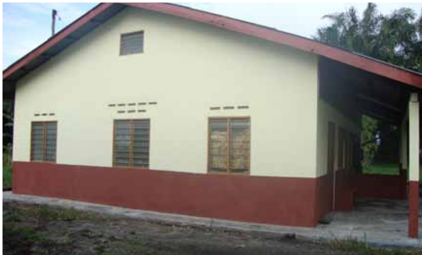
■ Housing - Refurbished Labour Lines, Teja Estate
